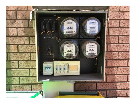
Figure 1 shows a typical shared residential switchboard/meter box. The switchboard/meter box configuration is too small to replace one existing meter with a smart meter let alone all meters. As a result, the entire meter board needs to be replaced (at considerable cost to either the retailer or the customer) before a smart meter can be installed.
